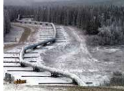
The Trans-Alaska Pipeline System was constructed between 1975 and 1977 to move oil from the oil fields of northern Alaska to the northernmost ice-free port of Valdez, Alaska. Eleven pumping stations maintain the oil flow along the 1,300 km pipeline, which can carry up to 2.1 million barrels per day.
